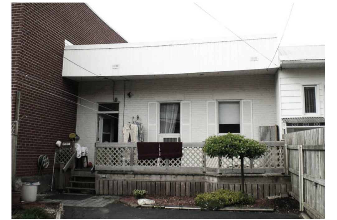
BACKYARD ELEVATION BEFORE THE RENOVATIONS
